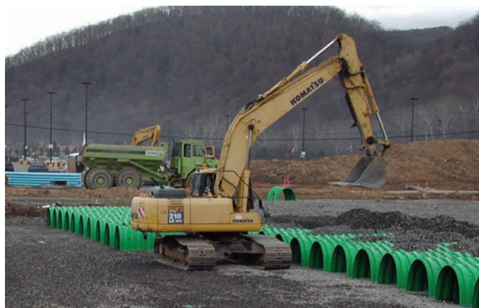
Installing embedment stone around chambers.
