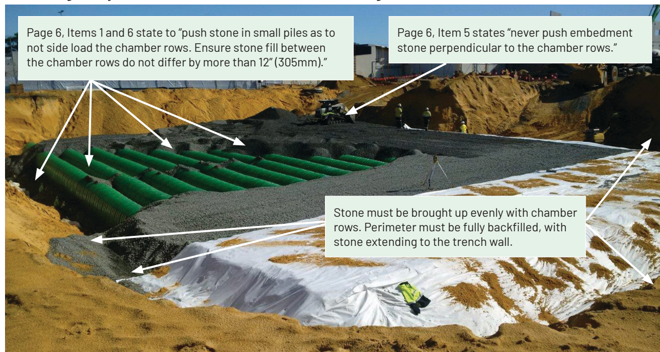
Non-recommended backfilling of system.
